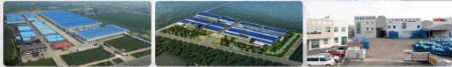
Wincell Insulation Manufacturing Center
